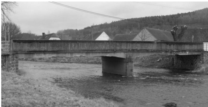
Fig. 1 Side view of analyzed bridge
